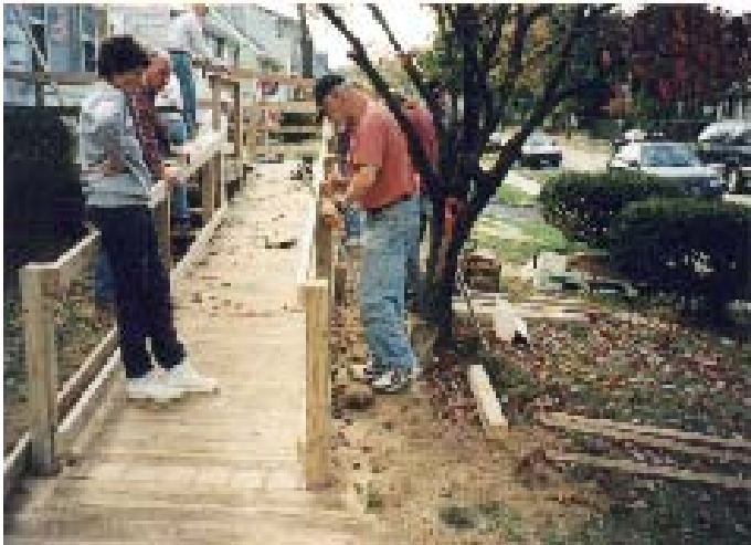
Volunteers building a wheelchair ramp
